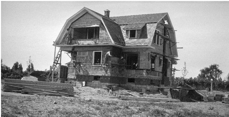
121 Corwin Rd. from rear - note streetlight at left
